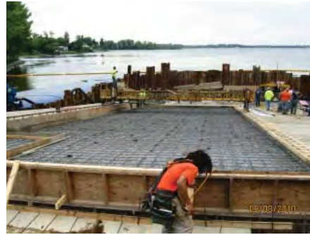
Installation of 3 lane launch ramp at City of Plattsburgh Boat Launch.
