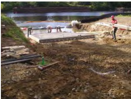
Installation of launch ramp at Rogers Island Pool Boat Launch.
