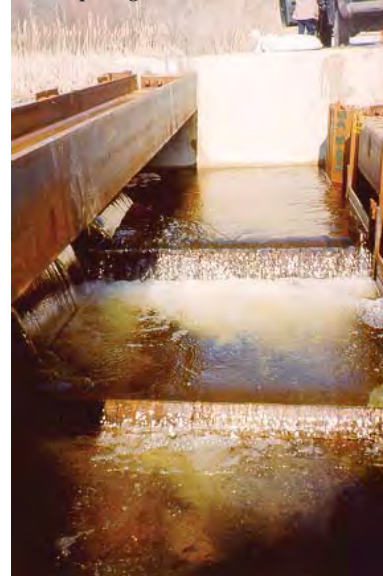
Fish passage structure on French Creek
